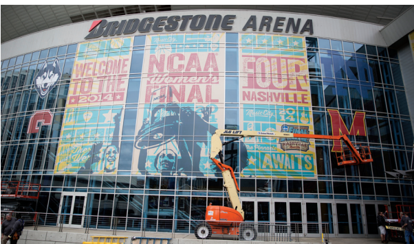
Bridgestone Arena perforated window vinyl
